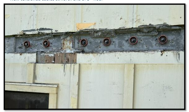
• New tensioned cables at south end of 3<sup>rd</sup> floor
