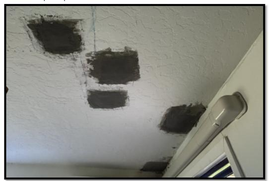
Spall repair at lanai soffit
